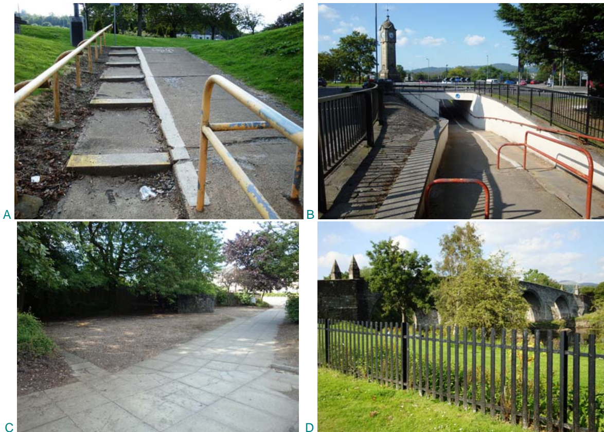
Fig 16A & B: underpasses in the surrounding area detract from the approach to the Stirling Old Bridge; C: open space adjacent to the Brig Haf tenement; D: heavy utilitarian fencing separating the riverbank and the walkway.
